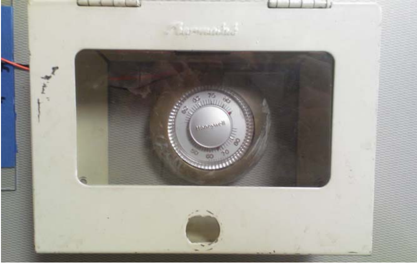
Photo of Box Alarm
