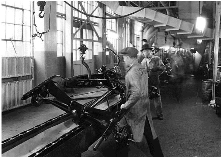
1933: Ford chassis assembly line
