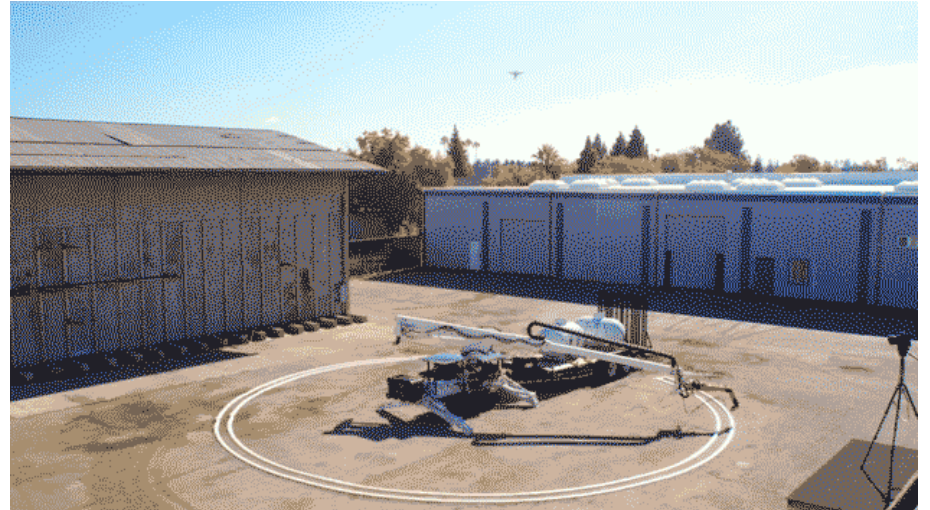
Robots 3D-Printing the house
